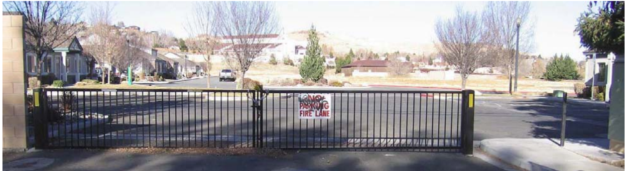
Existing Fence/Emergency Access/Pedestrian Access at Holman Way
